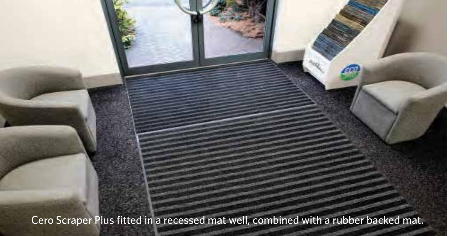
Cero Scraper Plus fitted in a recessed mat well, combined with a rubber backed mat.
